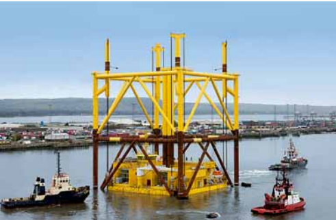
Tug boats pull a giant, floating switchgear structure to its destination. Such systems can convert up to 1 GW of electricity into highly efficient direct current.
