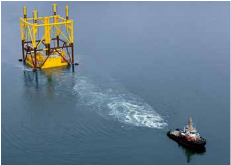
Tug boats pull a giant, floating switchgear structure to its destination. Such systems can convert up to 1 GW of electricity into highly efficient direct current.
