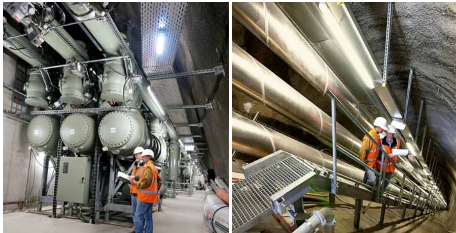
Gas-insulated transmission lines can carry high voltages in environments where masts are impractical.
